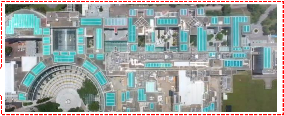
HKUST Launched the Largest-Scale Solar Power System among local universities, 2022 ( 8,000 solar panels, 50 locations on campus)
